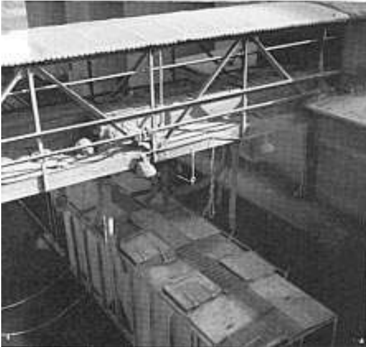
Loading bulk cement into a covered hopper car at The Universal Atlas Cement Company, Leeds, Ala - 1958
