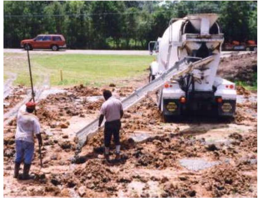
Unloading the Concrete on the job site
